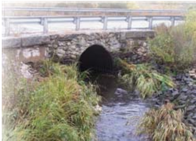
Culvert over Labor in Vain Brook, Somerset Brian Graber
